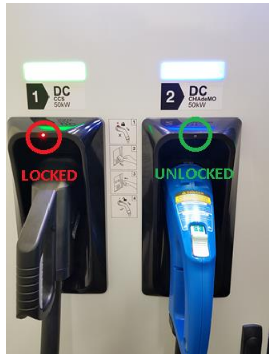
Figure 7. CHAdeMO Connector unlocked
