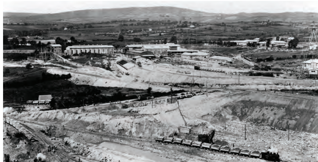
The powerhouse construction site in summer 1926. (Credit: Siemens AG, Munich/Berlin)
